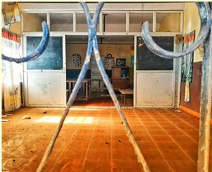
Inside the building before work began
