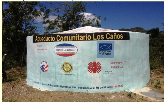
Aqueduct storage in Los Canos, Dominican Republic
