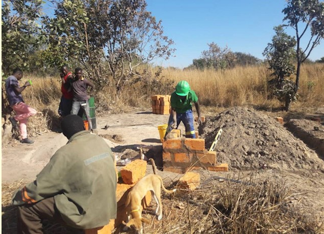
The first bricks
